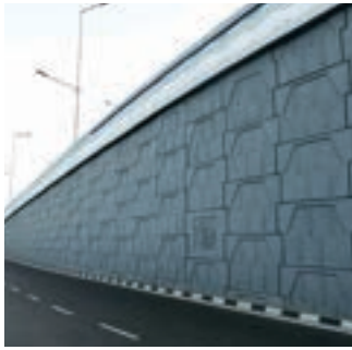
Retaining Wall Solutions
